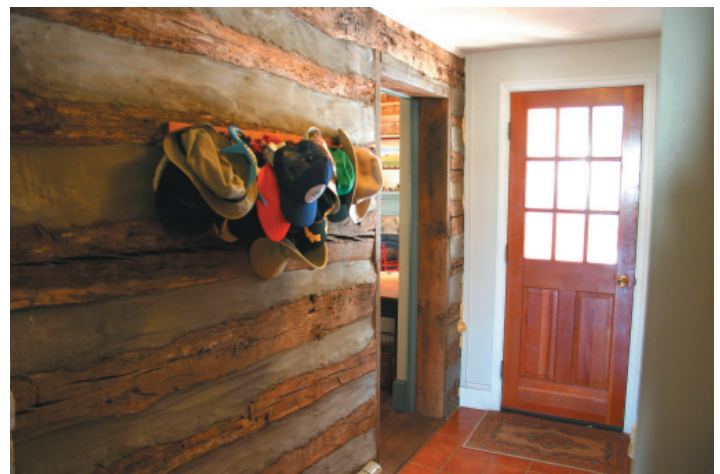
FIGURE 2-3. The log construction of the original structure may be seen where the exterior face of the west elevation is encapsulated in a modern addition.
