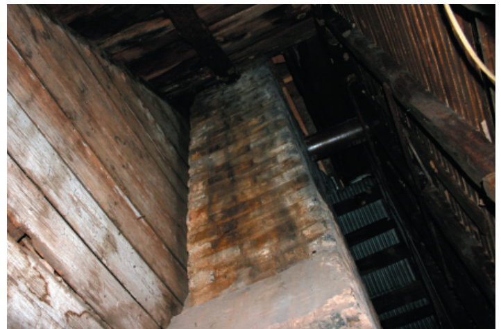
FIGURE 8-4. Chimney of period I house. The east gable of the Meeks House has been incorporated into the post Civil War addition, and is accessible from a storage area that serves as in-fill between the two buildings. Within this space, it is possible to examine the whitewashed masonry chimney and beaded weatherboard siding of the original house, as well as the hewn pole construction of the ca. 1870 addition.
