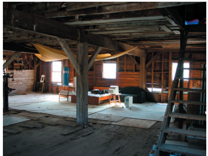
FIGURE 1-10. The second story viewed from the top of the stairs, facing southwest. The whitewashed ceiling joists and attic flooring are a mix of two periods, both recycled in the period III building. The exterior walls were sheathed on the inside with horizontal boards in the western portion of the second story; framing in the eastern half was left exposed.
