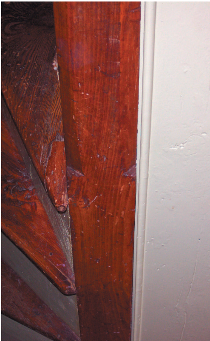
FIGURE 9-7. Stair detail. The enclosed winder stair wraps around a structural post that is handsomely chamfered.
