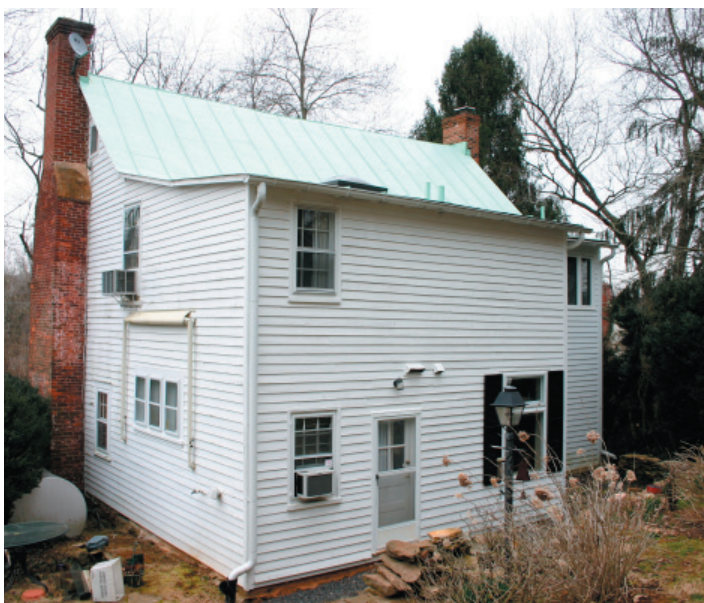
FIGURE 3-2. View from the northwest. The two-story rear wing probably dates to the 1850s reorganization of the house into a center-passage plan. The lower portion of the chimney at the left or north end dates to the 1790s, extended in the 1820s, and with a cap rebuilt in the 1970s. The south chimney was entirely built in the 1970s.
