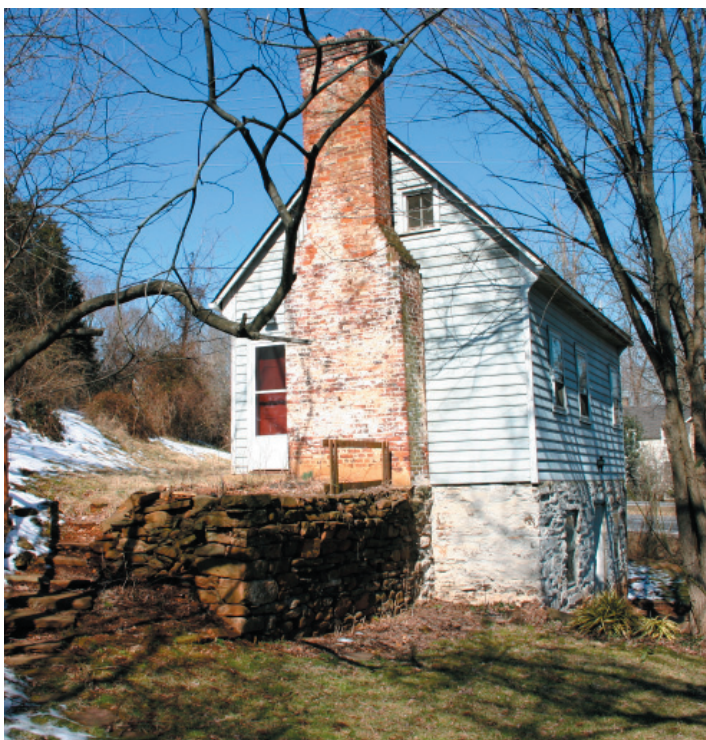
FIGURE 7-3. View from southeast. The stone and brick chimney serves fireplaces on the cellar and first floor. The door to the left of the chimney is probably not original, as it would have eliminated a key structural brace. Lee Highway and the Buckland Tavern are visible in the background.
