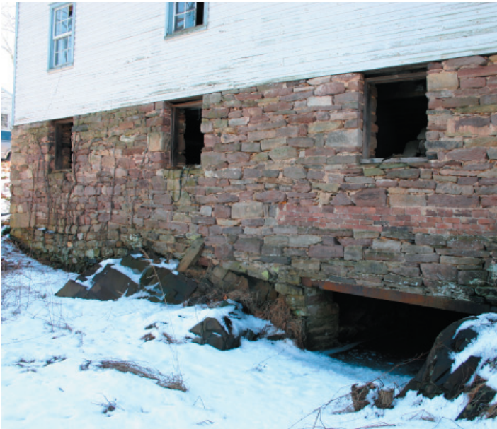
FIGURE 1-4. Stone foundation and tail-race portal, east elevation. The sills for the frame superstructure are recycled from the first-period mill, as demonstrated by a careful examination of the window openings. The bottom faces of the sills are exposed above these openings, and reveal hand-hewn surfaces and vacant mortises, indicating they have been recycled for this building.
