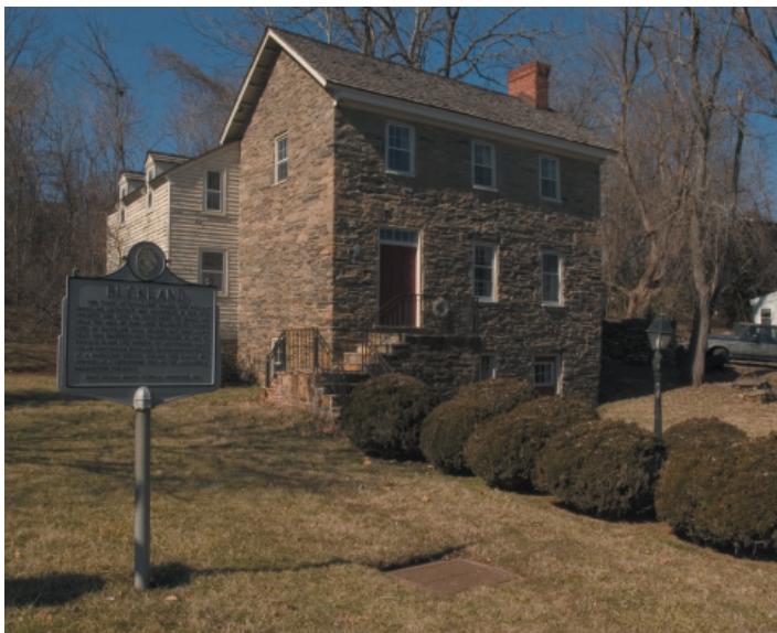
FIGURE 6-2. View from southeast. The stone steps were added in the late 1940s; the rear addition dates to 1975-76.
