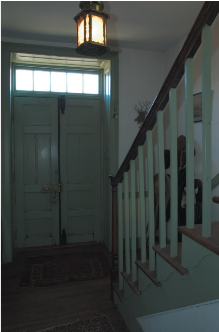
FIGURE 6-3. Entry passage and staircase, facing east. The pair of paneled doors at the front entrance are of the appropriate period for the house but are of oak construction, a rare occurrence in northern Virginia. Most likely they were salvaged from elsewhere and installed by Grace Bear in the late 1940s. The delicate newel post is typical of the 1810s and early 1820s.
