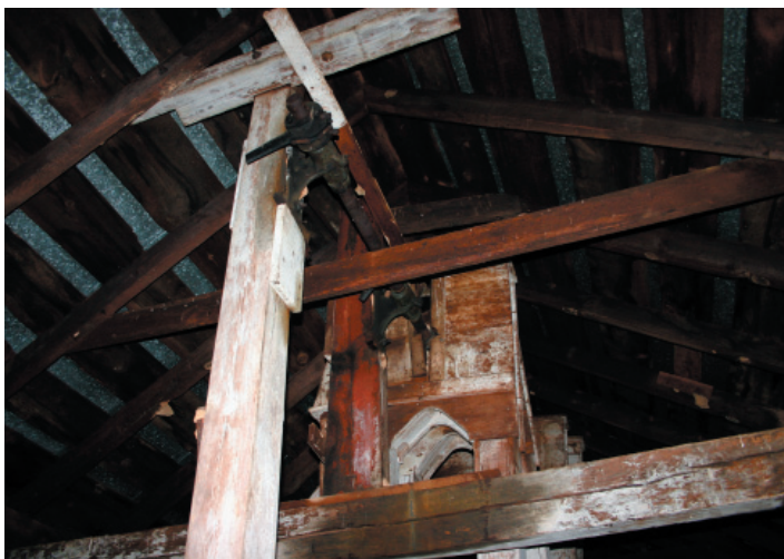
FIGURE 1-13. View of the north end of the drive shaft, which extended for most of the length of the third story. In this view, two iron pulleys have broken off, leaving remnants of the spokes. Note the mixture of framing material—hewn and whitewashed timbers from an earlier structure, and circular-sawn, unfinished rafters joined at the ridge with mitered and nailed joints rather than mortise-and-tenon joints.
