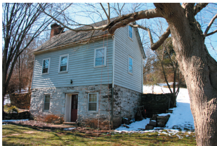
FIGURE 7-2. View from northeast. The stone retaining wall that projects from the north gable (to the right in this image) is a remnant of the hyphen that once joined the Trone House to the Stage Coach Inn, a building which faced the Warrenton Turnpike and was demolished in about 1935. Historic photographs indicate a two-story porch extended across the east or principal façade of the Trone House, with doors in the north and south bays of the first story, later altered to windows.
