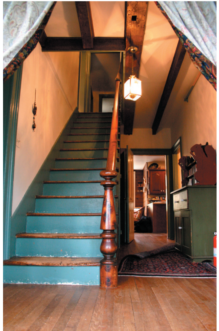
FIGURE 3-4. Front passage, facing west. In the 1850s, the interior partition was removed and the two-room plan was altered to a center passage with flanking parlor and dining room. The substantial ceiling joist visible to the right of the staircase served as a girt for the original partition. One mortise for the partition is visible in that beam and the base plate for the ceiling fixture conceals another. The present stair dates entirely to the 1850s, as suggested by the richly turned newel post and mid-century technological evidence.
