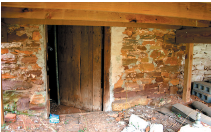
FIGURE 8-5. Cellar entry. Located at the west end of the south elevation, this doorway opens into a shallow, unheated cellar. Note the contrast between the exposed stone foundation at the west end of the foundation and the whitewashed stonework to the east, suggesting the size and location of an earlier and smaller porch predating the post Civil War addition.
