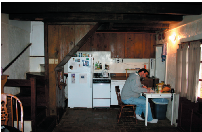
FIGURE 7-6. The cellar and stair, facing north. Originally, this space was probably partitioned into two rooms. The lower run of the cellar stair has been reversed to create enough room for utilities and a kitchen across the north end of the enlarged space.
