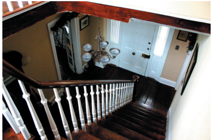
FIGURE 12-3. Staircase and passage. The stair rises against the north wall of the passage, originally serving a bedchamber to the south and an unheated chamber at the west end of the second-story passage. When the house was enlarged to the north, a second set of steps was added, rising to the north from the landing to a new bedchamber.
