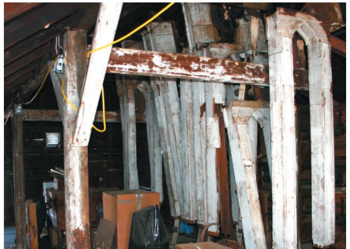
FIGURE 1-12. View of the third story, facing northeast. Wooden housings, painted white, served as a protective casing for the canvas conveyor belts that brought freshly-ground grain to the top of the mill. Originally, these would have extended all the way down to the cellar.
