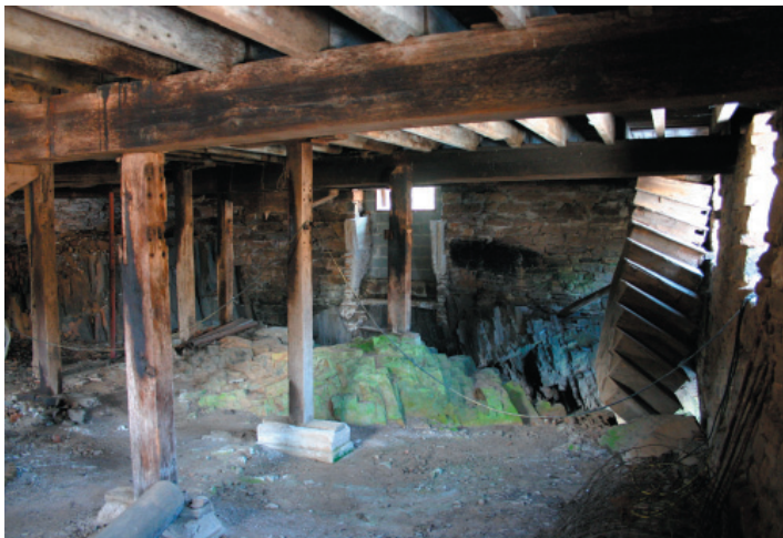
FIGURE 1-6. View looking north into the northeast corner of the cellar level, showing the wheel or turbine pit cut from stratified bedrock, and the partially collapsed stair to the first floor cantilevered across the pit. Water was delivered to the wheel or turbine through the opening at left (later reduced and converted to a window) and flowed out of the building through the portal under the stairs. Grease stains on the far wall, a chopped-out joist, and grease-stained vertical posts offer some clues to the location and alignment of the missing drive system.
