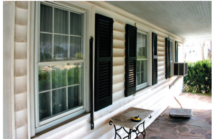
FIGURE 11-3. The windows flanking the front door on the west elevation retain hand-forged iron bars that could be placed across exterior shutters for security, a feature associated with commercial structures.
