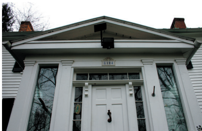
FIGURE 3-3. Detail of entrance porch. The entry porch was added in the 1850s when the interior plan was altered from two rooms to a center passage. In the 1970s the porch was enclosed and the Greek Revival door and sidelights were shifted from the main façade of the house to the front of the porch.
