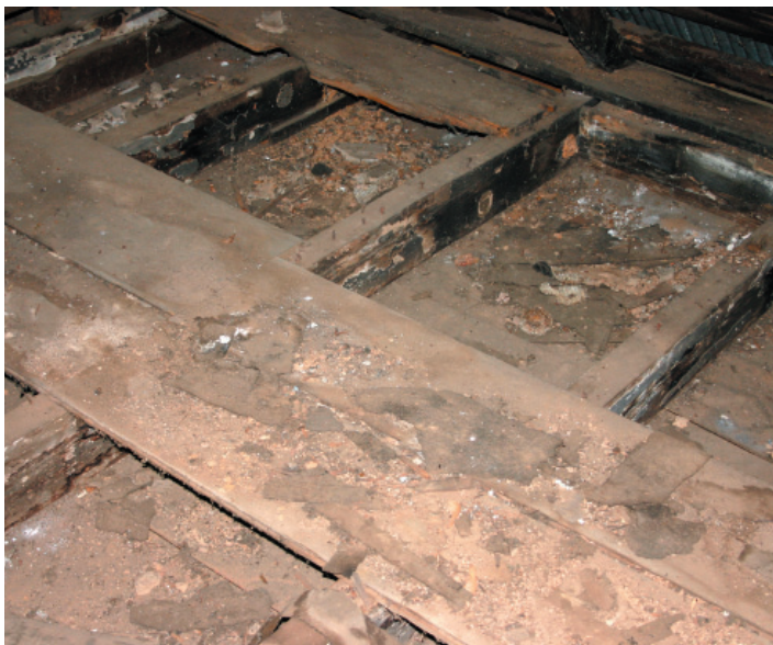
FIGURE 8-10. Garret flooring and framing. Random-width, tongue-and-groove flooring survives across part of the garret, secured with hand-forged T-head nails. Traces of whitewash and fireplace soot are evident on the first floor ceiling joists, which were exposed until the post Civil War period or later. The present ceiling is gypsum board, post-dating World War II.
