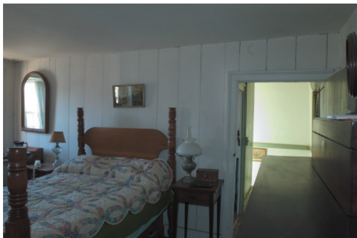
FIGURE 6-6. North bedchamber, second story, facing southeast. The second story is divided into a passage and two chambers by beaded vertical board partitions. At some point a door had been cut through this partition behind the smaller bedside lamp. This door opening was skillfully closed up with appropriate material in 1975-76.
