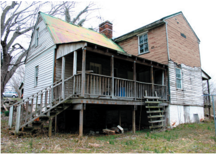
FIGURE 8-1. View from southwest. The original 16' by 16' one-room house (the left section in this view) was constructed by George Britton in about 1803, part of the development of an extensive tanyard owned and operated by Isaac Meeks from 1809 through 1824 or 1825. The two-story frame section to the east (right) was added sometime after the Civil War using hewn-pole construction in a local vernacular version of balloon framing.
