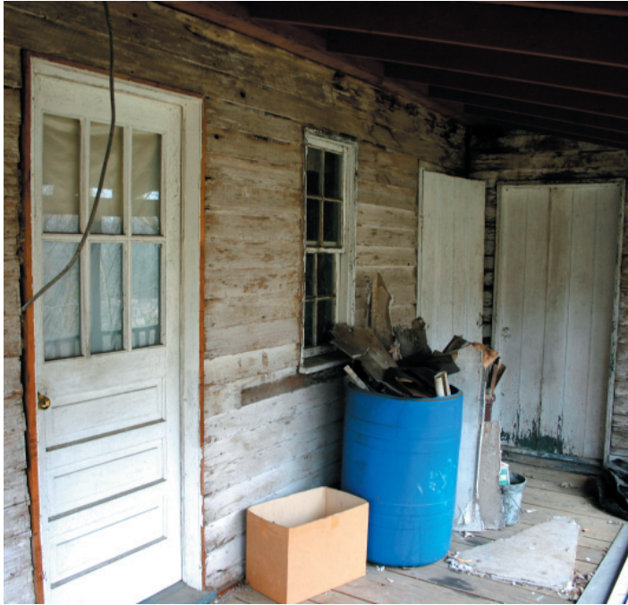
FIGURE 8-3. Detail of south elevation, protected by the rebuilt porch. The door in the left foreground opens into the 1803 house, while the door at the far end of the porch serves the post Civil War addition. A third door, partially concealed by the blue barrel, opens into a storage area, and reveals the masonry chimney and early beaded siding on the east end of the early house.
