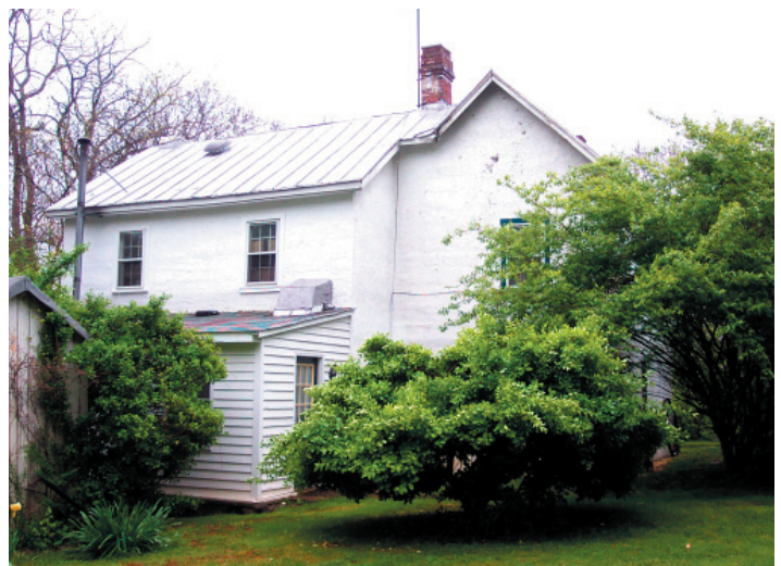
FIGURE 4-4. North elevation from the northwest. The original one-story log house is at left, concealed behind a 1970s lean-to addition. The outbuilding in the left foreground is a board-and-batten structure of about 1900 constructed over a root cellar or ice-house pit.
