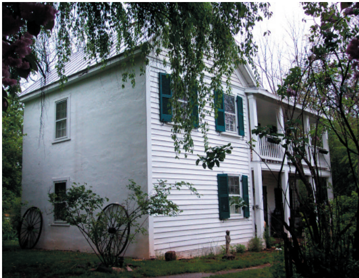
FIGURE 4-3. View from southwest. The west wing in the foreground was added around 1900 by “Bun” Graham, using a late form of hewn pole construction widely used in Buckland from the 1850s to about 1900. The stucco was added in the latter part of the twentieth century.
