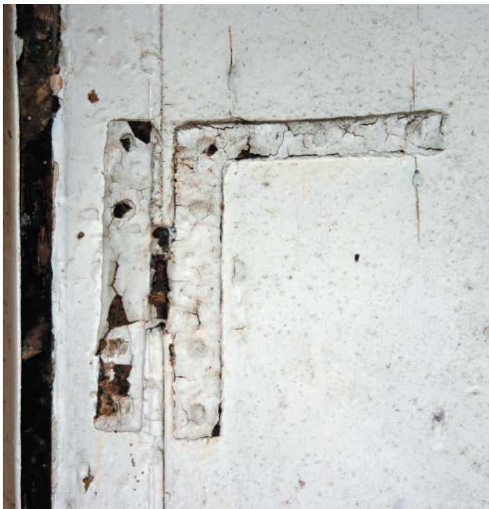
FIGURE 8-8. Door to winder stair. The beaded batten door is hung on 7" hand-forged HL hinges secured with hand-wrought nails.
