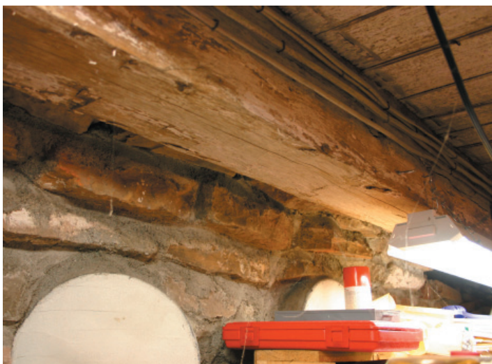
FIGURE 3-9. Cellar ceiling details. The original ceiling joists are hewn and pit sawn and the flooring is gauged and undercut. The stone foundation walls, joists, and the bottom face of the floor are whitewashed, an indication the cellar was used for storage, accessible through a bulkhead entrance near the north end of the rear or west wall.
