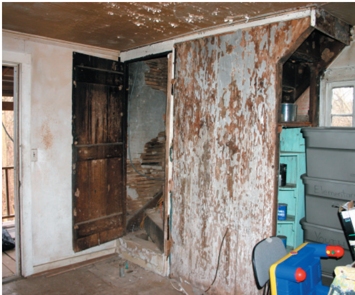
FIGURE 8-7. Stair in southwest corner of period I house. A tightly proportioned winder stair provides access to the garret of the original house. The plaster within the stair enclosure is applied to circular-sawn lathing, an indication of improvements made after 1850, most likely when the east addition was constructed ca. 1870.
