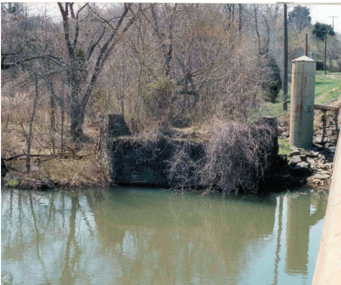
FIGURE 12. Stone bridge abutment at Broad Run, Buckland. This abutment dates to the construction of a timber bridge across Broad Run in 1808, and later served as the support for an iron bridge built in 1890 and replaced in 1927. The road bed of the early turnpike survives for approximately 70 yards to the west of the abutment. Buckland Preservation Society, 2004.
