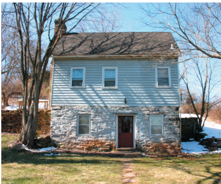
FIGURE 7-1. East elevation from Buckland Mill Road. This frame house on a full stone cellar story was built by blacksmith and lay preacher John Steadman Trone about 1825.
