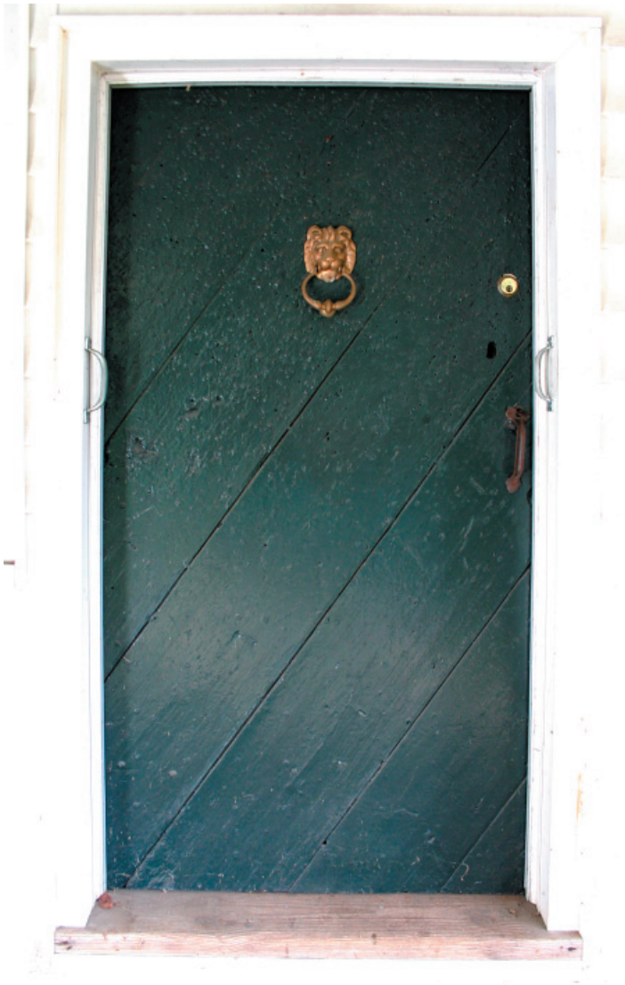
FIGURE 11-2. Principal entrance door: An unusual feature is the original double-layer door, with beaded boards laid diagonally on the exterior face and vertically on the interior. The upper part of the door bears the scars of hundreds of tacks used to post public notices on a building that is believed to have served in the nineteenth century as the town post office.
