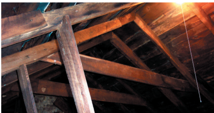
FIGURE 4-9. Roof framing in period II attic, facing west. The 1½-story log house was raised to two stories shortly after the Civil War. The new roof was framed with circular-sawn common rafters, mitered at the ridge and nailed with mature machine-made nails. Circular-sawn collar pieces were scabbed on at a later date using wire nails, which came into use in the 1880s.
