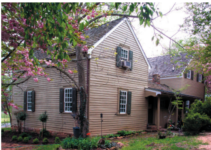
FIGURE 9-1. View from northeast. The early house is a “true” story-and-a-half, in which the wall framing extends up into the garret story, providing more space and eliminating the need for kneewalls. A rebuilt one-story wing now serves as a hyphen to the 1980s addition in the back-
