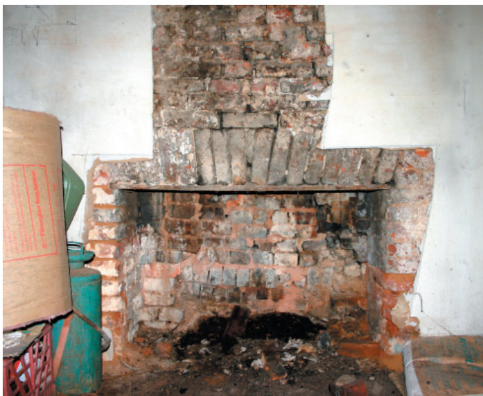
FIGURE 8-6. Fireplace, first floor of period I. The fireplace is smaller than would be expected for a chimney of this size, but the exposed portion of the chimney shows no evidence of alterations.
