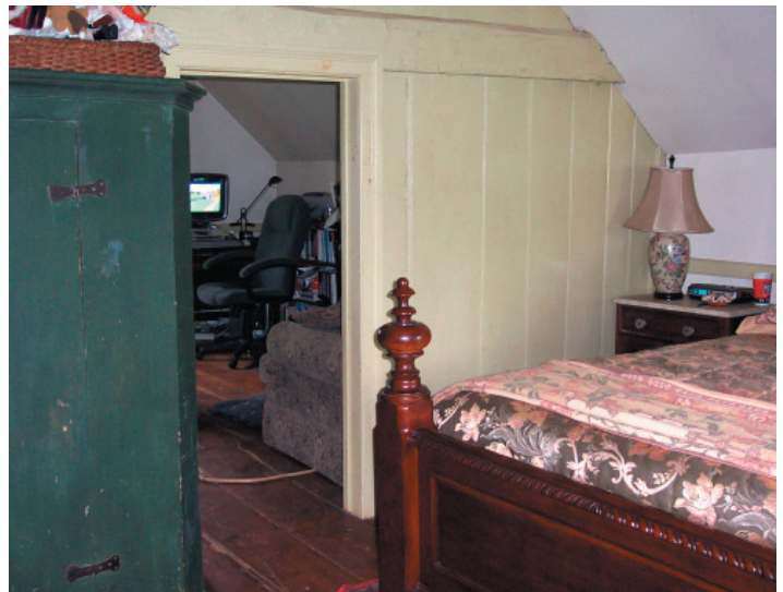
FIGURE 9-8. Second-story partition and tie beam from south bedchamber. The substantial tie beam visible just above the door serves as an important structural member. It is secured to a pair of rafters that are more robustly proportioned than the rest of the roof, providing added strength near the center points of the side walls. The partition between the chambers is constructed with beaded vertical boards that range up to 16" in width.
