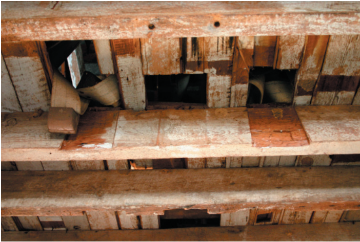
FIGURE 1-11. The second-story ceiling is framed with joists recycled from an earlier structure and overlaid with recycled flooring as indicated by the ghosting of a different joist system captured by the whitewash. Boxed, square-section chutes delivered the grain from sifters and graders on the third story to machinery and storage bins on the first and second stories. The broad, shallow notches in the side of a joist in the middle of this view are evidence of the boxed elevator conveyors that carried freshly-ground grain to the top of the building to begin the gravity-fed procession through sifters and graders.
