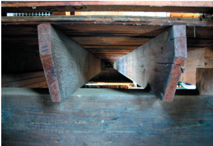
FIGURE 1-9. Floor joists for the second floor run continuously the full 40-foot length of the building from north to south. Note the tongue-and-groove flooring of the second floor and the complete absence of diagonal bridging to provide lateral stability to the joists, a feature that comes into practice in the mid nineteenth century for even the most routine domestic construction.
