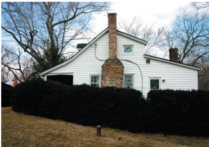
FIGURE 11-4. South elevation. The southern ten feet of this structure and the southern portion of the east lean-to (on the right in this image) date to a mid nineteenth-century expansion. The chimney dates to that expansion and serves a single fireplace on the first floor—the chamber above is unheated.
