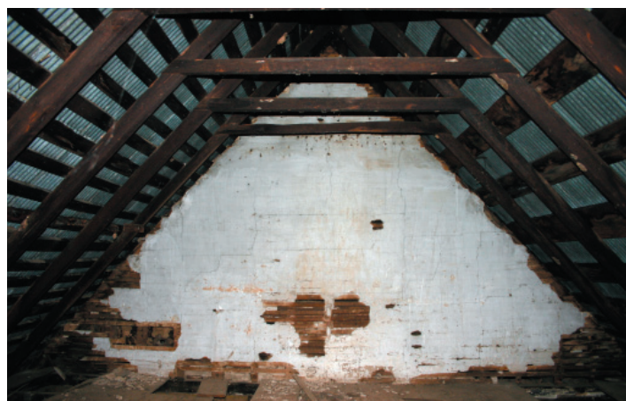
FIGURE 8-9. View of garret, facing east from the top of the stairs. The loft was floored but otherwise unfinished initially. Sometime after 1850, the gable ends were plastered all the way to the peak of the roof using circular-sawn lathing applied with mature cut nails. Even with this improvement, the roof frame was not upgraded with either whitewash or plaster. The sash-sawn, common-rafter pairs are set at 48 degrees, half-lapped at the ridge and nailed with hand-forged nails. Each pair is reinforced with an original collar tie, half-lapped and nailed to the rafters with hand-forged nails. Original nailers for a wood shingle covering survive on the north (left) plane of the roof but have been replaced to the south.
