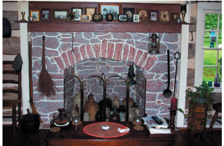
FIGURE 4-6. Fireplace on west wall of original house. The size of the fireplace opening indicates it was intended to heat this, the best room, but was not intended for cooking.
