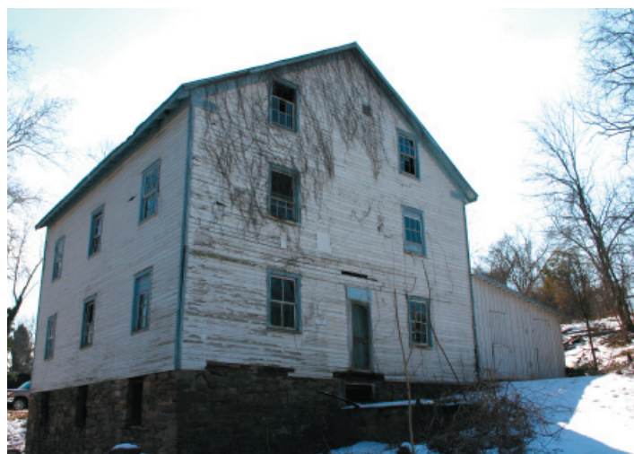
FIGURE 1-2. View from Northeast. The mill race arrived at the mill at the right margin of this photograph and was carried by a flume to the portal directly below the door in the center of the north gable elevation.
