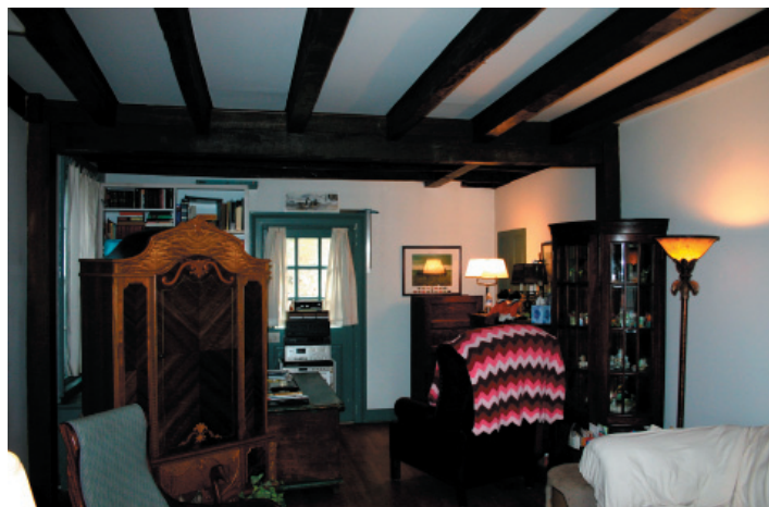
FIGURE 3-6. South parlor, facing west. In the original, two-room plan, the south room extended several feet farther to the north or right, and the original stair was probably located in the back right corner of this, the larger of the two rooms. In the 1850s, this room was reduced in size to accommodate the new, center stair passage. In 1976 the rear wall was removed and the room was expanded into the enclosed first story of a two-story rear porch.
