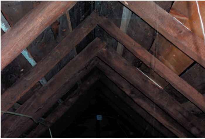
FIGURE 9-9. Roof construction. The common rafter roof is constructed with hewn and pit-sawn rafters set at 40 degrees and joined at the ridge with pinned mortise-and-tenon joints. The gable studs are riven from hewn stocks, mitered and nailed to the gable rafter pairs with machine-headed cut nails.
