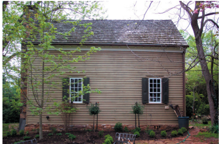
FIGURE 9-2. East elevation. Framing evidence indicates the north (right) window marks the location of the original front entrance, which opened into a generously proportioned stair passage to the north with adjoining parlor to the south. The restored nine-over-six windows are based on sash found in the south bay of the west elevation.
