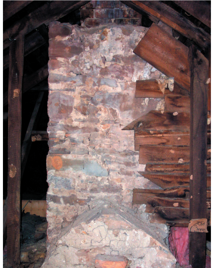
FIGURE 4-8. Original chimney viewed from the attic, facing west. The stone chimney with red limewash finish retains a clear outline of the pitched roof of the original 1½-story house, now encapsulated within the attic of the raised, two-story house. The shaft was extended in height with brick construction when the roof was raised, and the chimney received additional protection when the two-story west wing was added around 1900. Gable framing and siding from the period II west gable is evident to either side of the chimney. The attic beyond the chimney serves the west wing.
