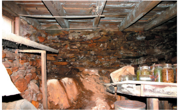
FIGURE 8-11. View of cellar, period I. The cellar provides just 4'-10" of clearance, and was never heated, indicating it was used for food storage rather than as domestic space. The flooring overhead varies considerably in thickness and has been gauged with a drawknife and undercut by as much as 1½" at the joists.
