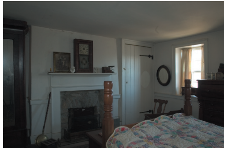
FIGURE 6-5. North bedchamber, second story. The best bedchamber is heated with a fireplace on the north wall. The fireplace surround is similar to the first-floor mantel, with Federal and Greek moldings. The wardrobe to the left of the chimney conceals an original window in the north wall.
