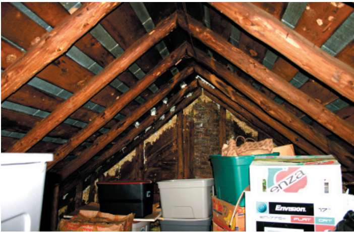
FIGURE 12-6. Attic of the main house, facing south. The roof is constructed of barked poles hewn flat on top, mitered at the ridge and nailed with mature, machine-cut nails. This roof closely matches the roof of the Buckland Church, and may also be the work of Leslie Sanders and Thurston Brown, who signed the church roof in 1856.
