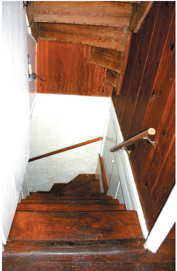
FIGURE 7-7. View of cellar staircase from first-floor passage. The lower run of the cellar stair has been altered, but the upper run, the flanking partitions and the stair to the garret are original.
