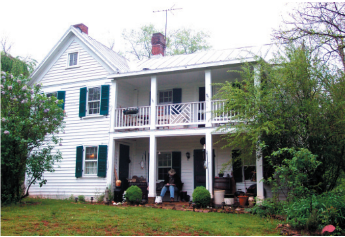
FIGURE 4-1. South elevation. The core of this house is a one-story log structure constructed by blacksmith Richard Gill by 1796. Gill’s house forms the first story of the right-hand section in this view. The house was raised to two stories shortly after the Civil War and expanded by the two-story frame addition to the left around 1900.
