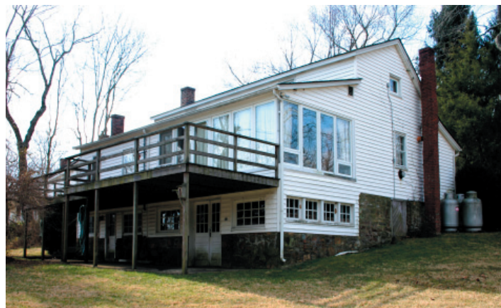
FIGURE 11-5. View from northeast. Lean-to additions conceal much of the east elevation, facing Broad Run. The southern portion of the lean-to (to the left) dates to the 1850s while the northern part was added in the 1970s.
