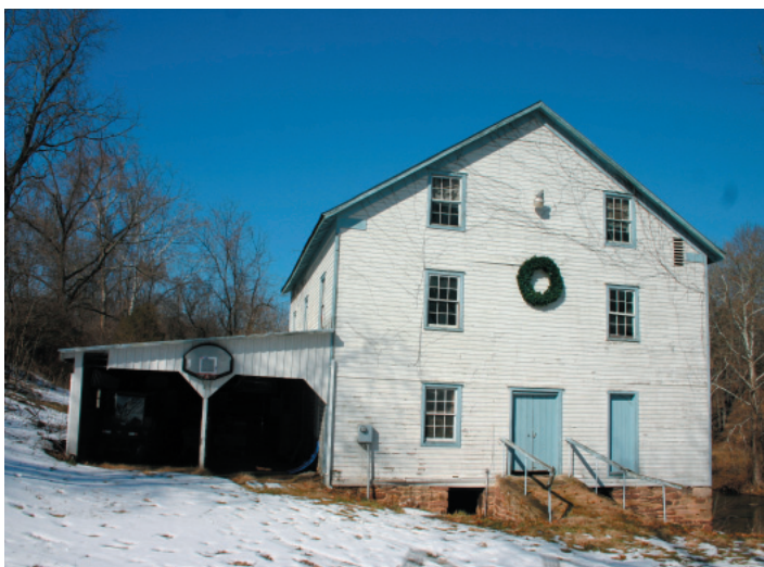
FIGURE 1-1. South Elevation. Broad Run is visible to the right of the building, and the mill race followed the tree line behind the lean-to shed, bringing water from a dam that was located about one-quarter mile upstream. When the light strikes the building at a raking angle, it is possible to make out promotional advertising stenciled onto the siding between the second-story windows, now covered by white paint.
