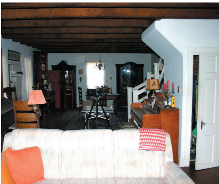
FIGURE 11-6. First-floor interior, facing north. The interior plan originally consisted of a heated counting room to the south and an unheated commercial store to the north. In the mid-nineteenth-century, the building was extended an additional ten feet to the south, and an outshut was added to the east. In 1953, Martha Leitch opened up the plan, exposed the ceiling joists, and rebuilt the stair.
