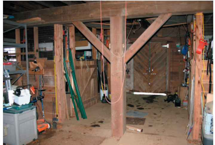
FIGURE 1-8. View from the center bay of the first floor, facing south to the double doors. The quadrants on either side of the entrance aisle were enclosed with horizontal planks and turkey wire sometime prior to 1973 for use as horse stables. Note the diagonal double-planked doors, tightly laid sheathing on the exterior walls, and the finely crafted timber framing.
