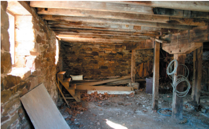
FIGURE 1-7. View of the south bay of the cellar, facing west. The chamfered post and massive bearing plate to the right are recycled from the earliest of three construction periods that can be identified in the mill.
