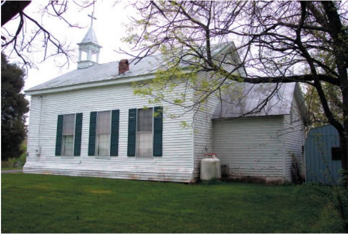
FIGURE 10-3. The bell cupola and the frame projection at the south end of the sanctuary are later features, probably added in the late nineteenth century, or perhaps in 1907, when the building passed into use as an Episcopal chapel.
