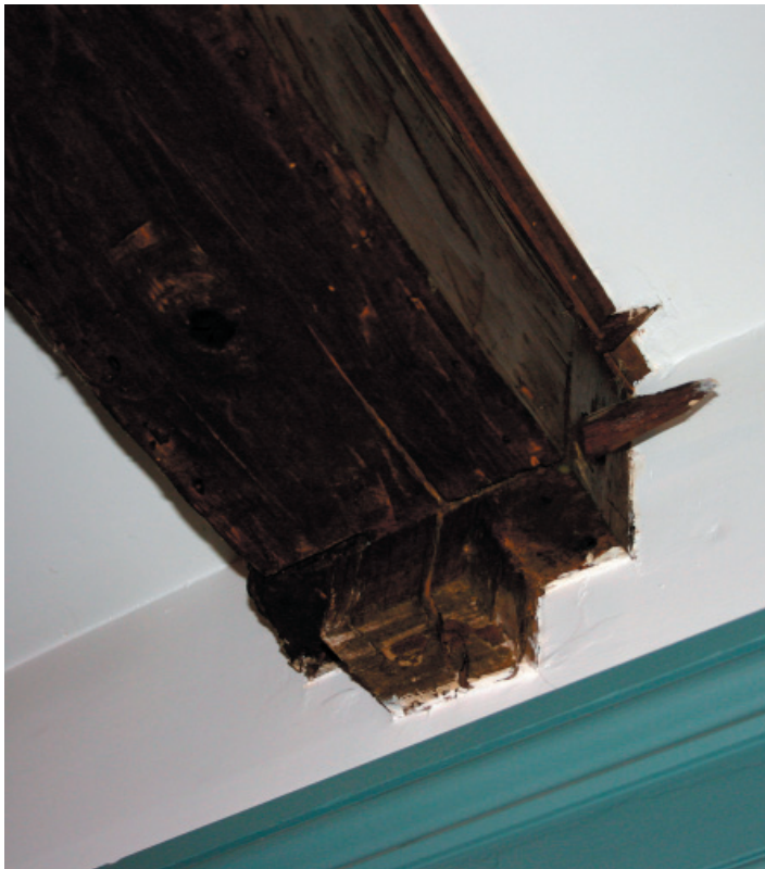
FIGURE 3-5. Detail of framing, ceiling of passage. The original structure was constructed with L-section corner posts and T-section intermediate posts framing the junction of the interior partition with the outside walls. When the two-room plan was altered to a center-passage plan in the 1850s, the original interior partition was removed and the T-section posts were chopped out to make way for the new front and rear doors. In this view, the truncated upper end of the T-section post in the west wall is evident above the rear door, still pinned to the girt that served to frame the interior partition.
