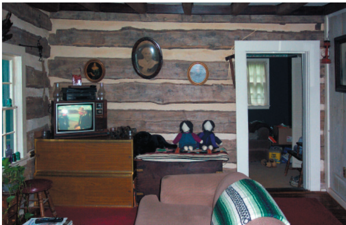
FIGURE 4-5. West parlor in the original house, facing north. The log construction is exposed on the north and west walls of the west room, as are hewn and pit-sawn ceiling joists. The partition to the right is constructed of beaded vertical boards, some early and others added as part of a late twentieth-century renovation.
