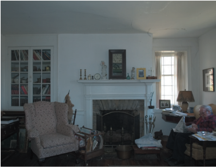
FIGURE 6-4. First-floor parlor, facing north. The parlor mantel is original and mixes Federal and Greek moldings in a fashion typical of the 1810s and early 1820s. The cupboard to the left retains original paneled doors below and is fitted with glass doors of the period salvaged from another house, but with muntins that align perfectly with the original shelves. The lack of a window opening in the west (left) wall indicates an original wing, and the lack of a door implies a desire to segregate the parlor from the rear wing—evidence that supports the likelihood this building was intended as a tavern.
